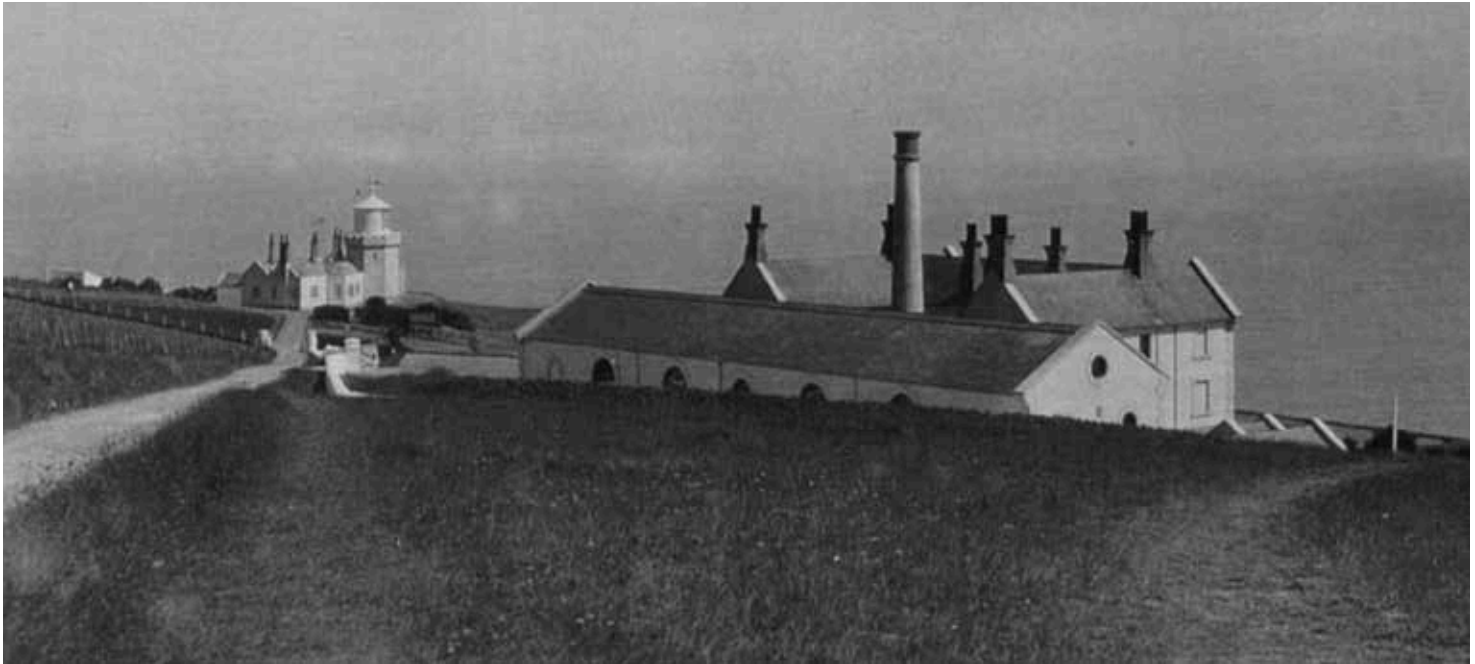
ABOVE: The engine house construction took place from 1869 to August 1871. It was a large facility, running left to right in the centre of the photo, and was designed to house the numerous magneto-electric generators selected for test. The tall chimney indicates that steam plant was also required to power the generators. The new office and accommodation two-storey house are on the far side, nearest the sea. The Low Lighthouse can be seen on the left; the High Lighthouse is behind the camera. Electricity from the chosen generators was sent to both High and Low lighthouses (the matrix of combinations is shown on p226) and the intensity of light produced by each was compared from the THV Galatea some 11.5 mi distant in the English Channel.
