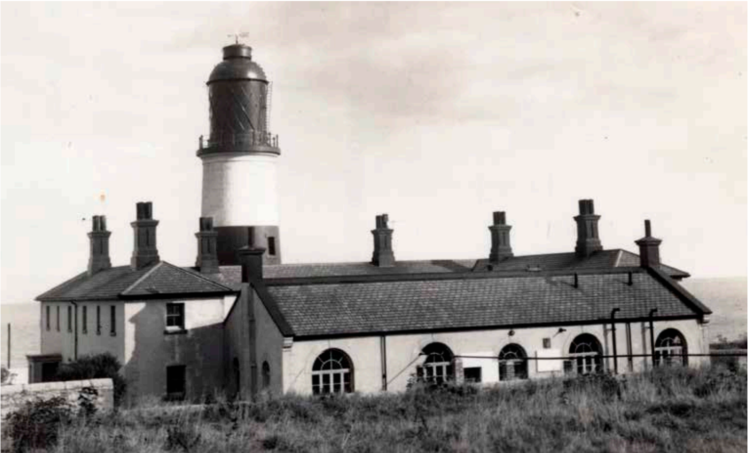
ABOVE: The lighthouse at Souter Point, Marsden - between Sunderland and South Shields. Following trials at both South Foreland (1859) and Dungeness (1861), it was built as the first fully electric lighthouse and lit on 11 January, 1871. The electric generator designed by Holmes that was installed at the time is preserved in the Science Museum (see p141).
